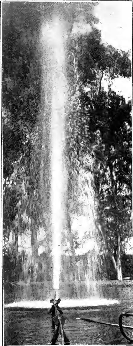
PUMPING WATER BY CONDENSED AIR. (Near Tulare.)
